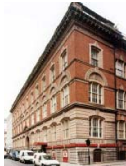
The Albany, Old Hall Street © English Heritage
